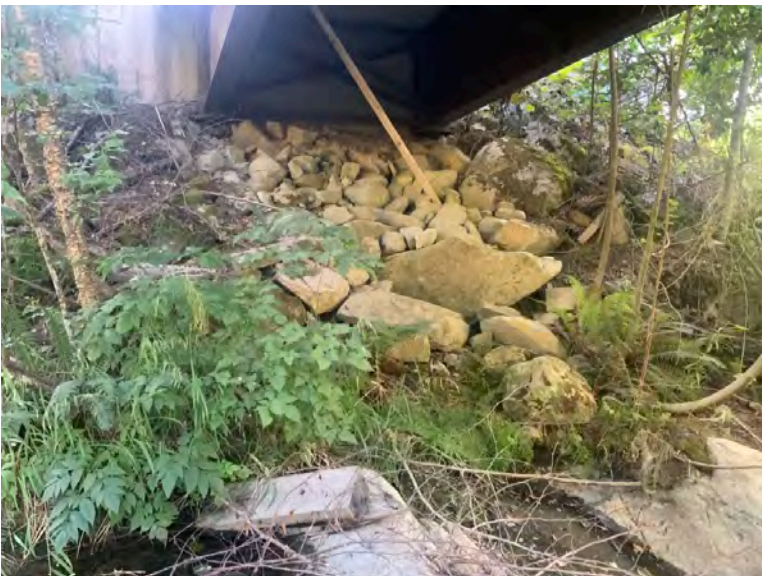
Left Bank Abutment when facing downstream
