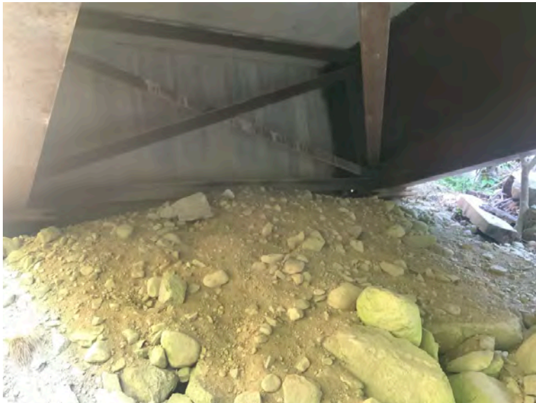
Right Bank Abutment when facing downstream
