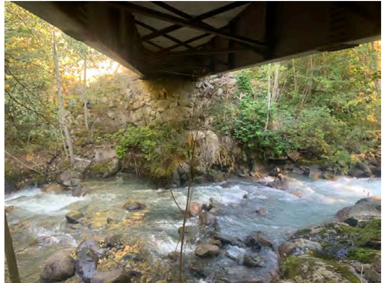
Right Bank Abutment when facing downstream
